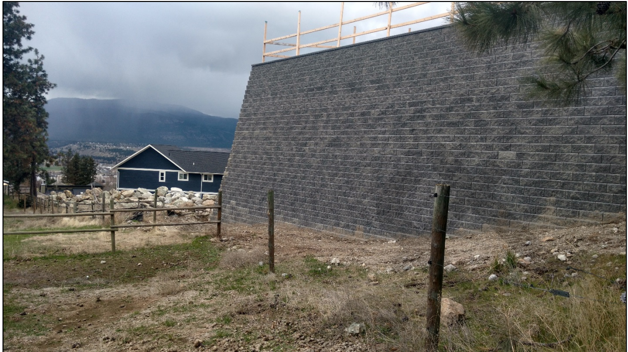
Figure 6: South Elevation looking west
